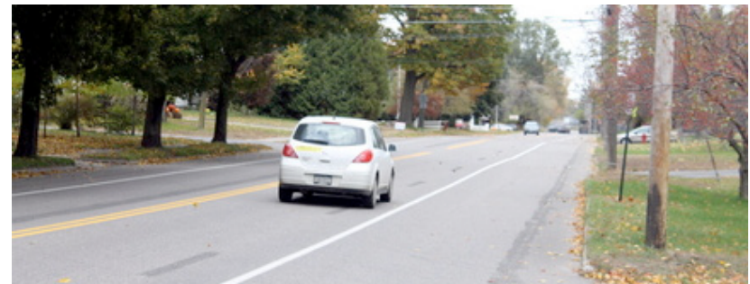
Elm Street after a "road diet" eliminated an unnecessary third travel lane .
