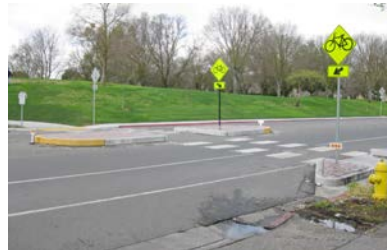
These raised islands provide a space in the median, protected by curbs, for pedestrians to wait for traffic while crossing a busy or wide, multi-lane street.
