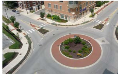
A roundabout at a major intersection with a sloped truck apron and a center planting island.
