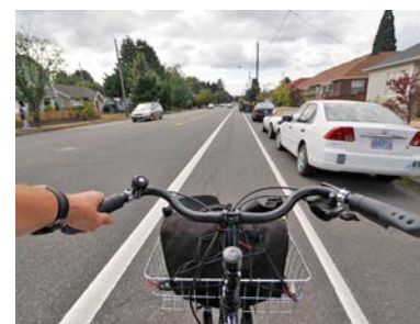
Bike lane located between travel lane and on-street parking lane. One hazard of a bike lane adjacent to on-street parking is the possibility of a car door being opened in front of an oncoming bicycle. The bike and parking lanes should be wide enough to allow vehicle doors to be safely opened and bicyclists room to maneuver.
