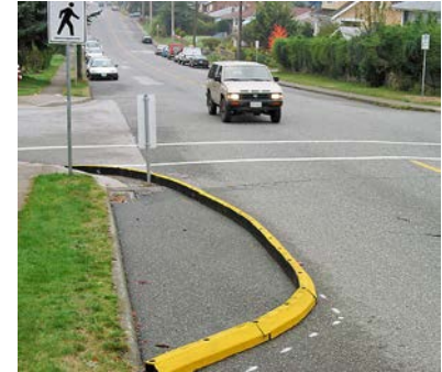
A temporary curb extension.
