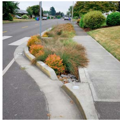
This curb extension on a residential street has multiple purposes. It narrows the crossing for pedestrians and is attractively landscaped. It also collects, filters and infiltrates stormwater.
