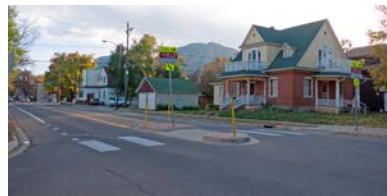
These raised islands provide a space in the median, protected by curbs, for pedestrians to wait for traffic while crossing a busy or wide, multi-lane street.
