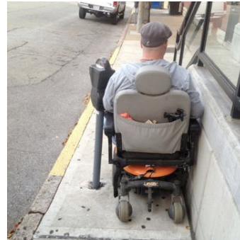
Sidewalk too narrow for wheelchair.
