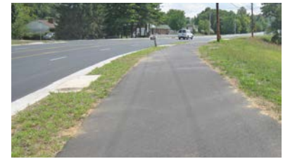
Paved shared-use path adjacent to the road in place of a sidewalk.
