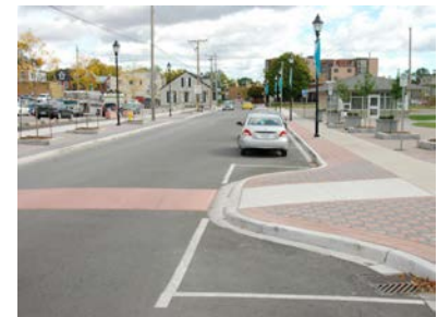
This curb extension is constructed with concrete pavers and is part of the overall streetscape design on this commercial street.
