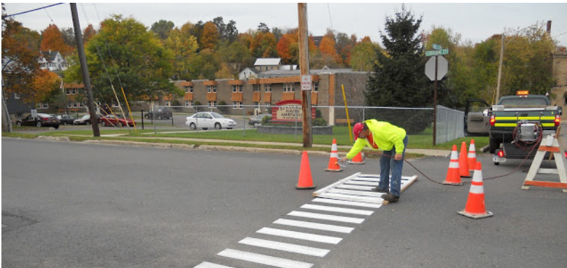
Crosswalks being painted on Catherine Street.
