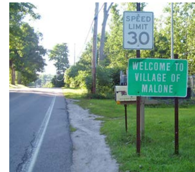
This paved shoulder is not wide enough to safely accommodate bicyclists.
