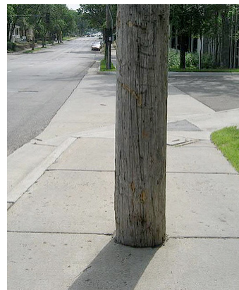
Utility pole blocking sidewalk.
